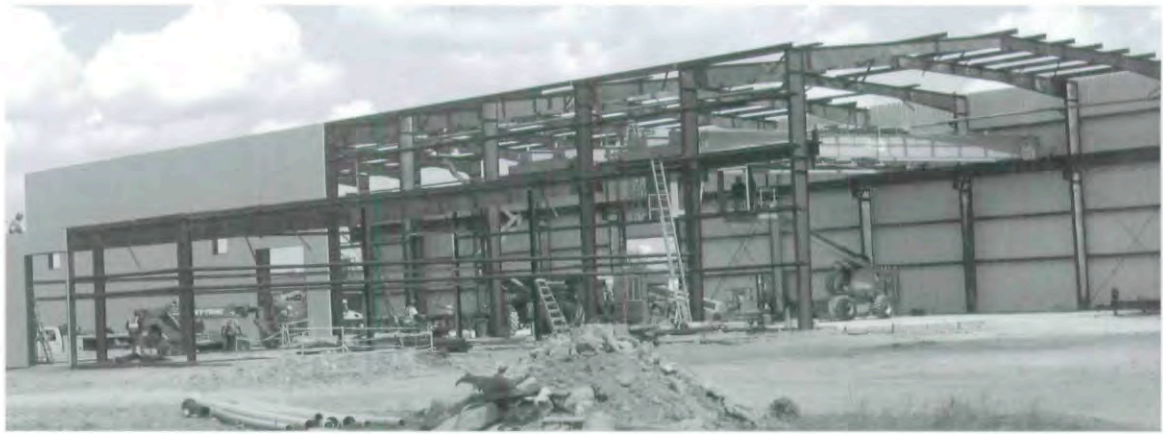
ShawCor Pipe Protection – new building expansion.
